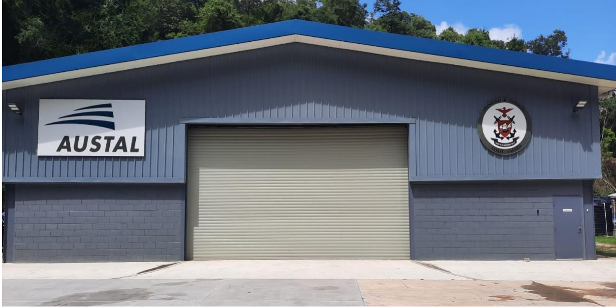
Caption: The new AUSTAL Maintenance Facility of the Trinidad and Tobago Coast Guard, located at Trinidad and Tobago Coast Guard, Hart's Cut Base, Chaguaramas. The facility was handed over at a ceremony on Tuesday October 17, 2023
